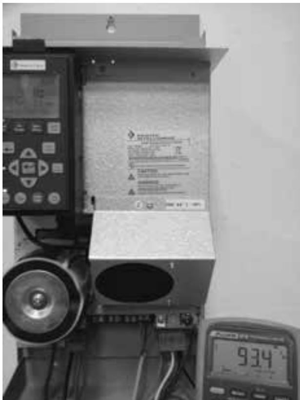
**Figure 20. 3 phase 30Hz voltage measurement**
