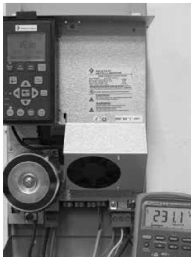
**Figure 19. 45Hz voltage measurement w/out LPF**
